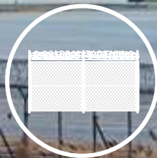
Perimeter Intrusion Detection
